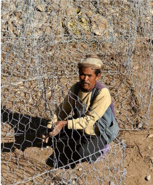
Using gabion cages (bio-engineering) to protect against landslides in Charnawati, Nepal
